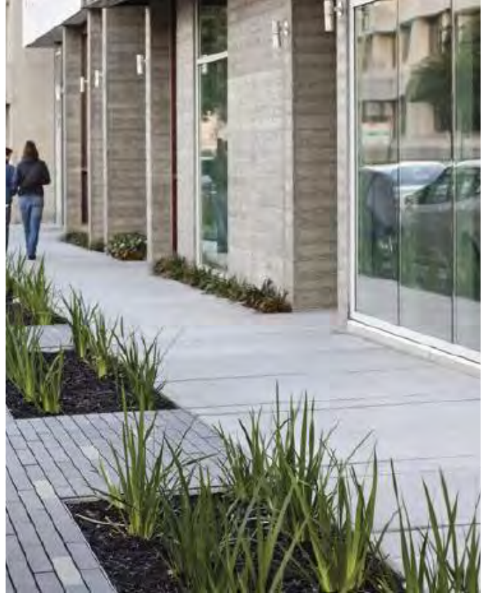
Stormwater areas and porous pavers
