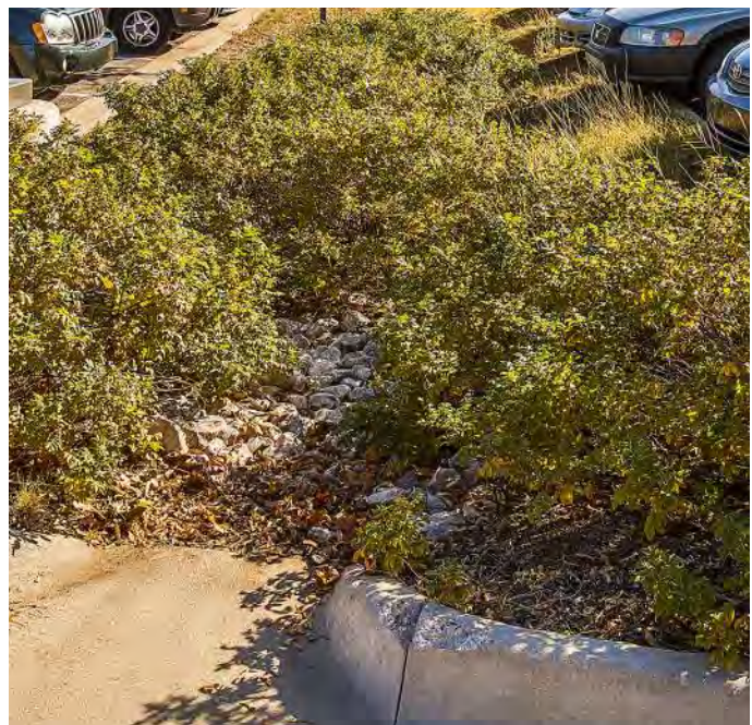
Rain Garden Parking Lot Island
